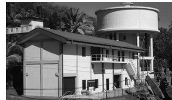
Greater Kandy Water Supply Scheme
