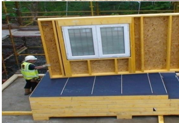
Figure 1 (c): Timber frame panel (closed type)
