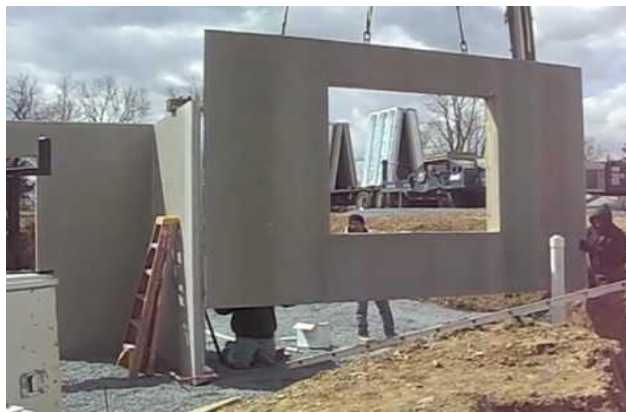
Figure 1(a): Precast concrete wall panel Figure 1(b): Light weight steel frame panels
