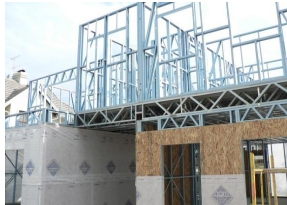
Figure 1(a): Precast concrete wall panel Figure 1(b): Light weight steel frame panels
