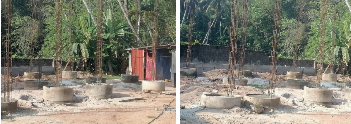
Figure 5.2: Implementation of Precast Cylindrical Rings with RCC Cages & Column Reinforcements, Foundation Designed by the Researchers (Construction Site B)
