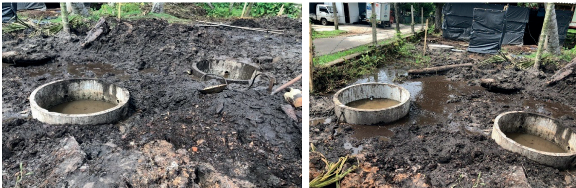
Figure 5.1: Implementation of Precast Cylindrical Rings with Filling Quarry Dust, Foundation Designed by the Researchers (Construction Site A)
