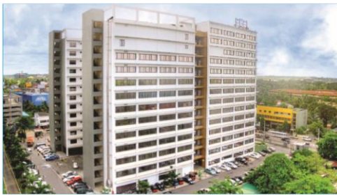
Sethsiripaya Administrative Complex - Stage II
