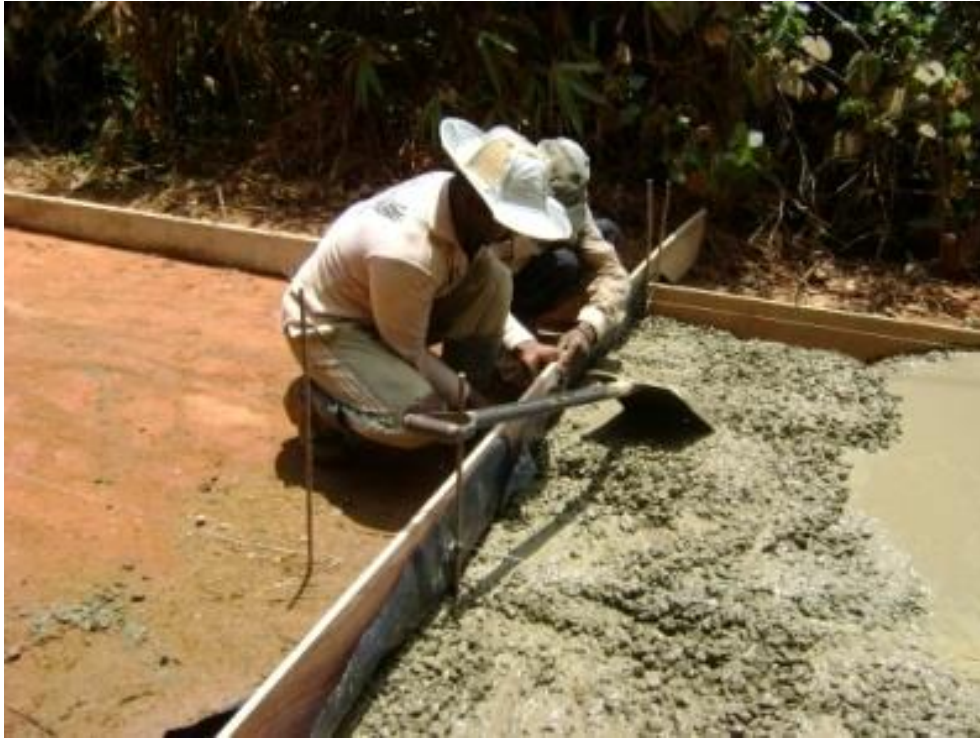
Figure 04: Construction of Half Depth Contraction Joint
